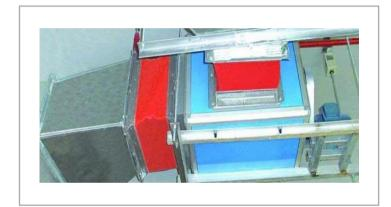
In order to isolate vibrations and noises caused by air handling units, fans or other equipment connected to air ducts, it is highly recommended to install a flexible duct connector joint between the outlet of these devices and the air duct.
